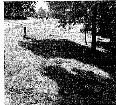
Figure III-3: Existing Sidewalk near Cove Lane Intersection
