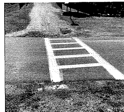
Figure II-4 – Water Street Crossing
